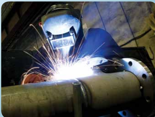
Skilled and experienced welders with a 99% or greater weld acceptance rate.
