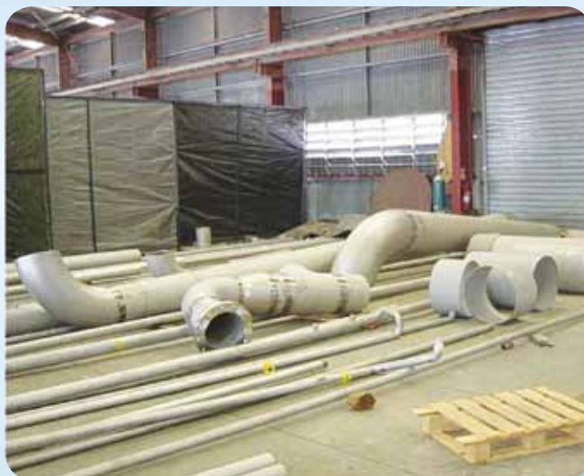
Rapid response shop and field fabricated spool capabilities and laydown acreage.
