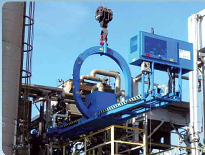
Aerial extractor pulling an exchanger bundle.
