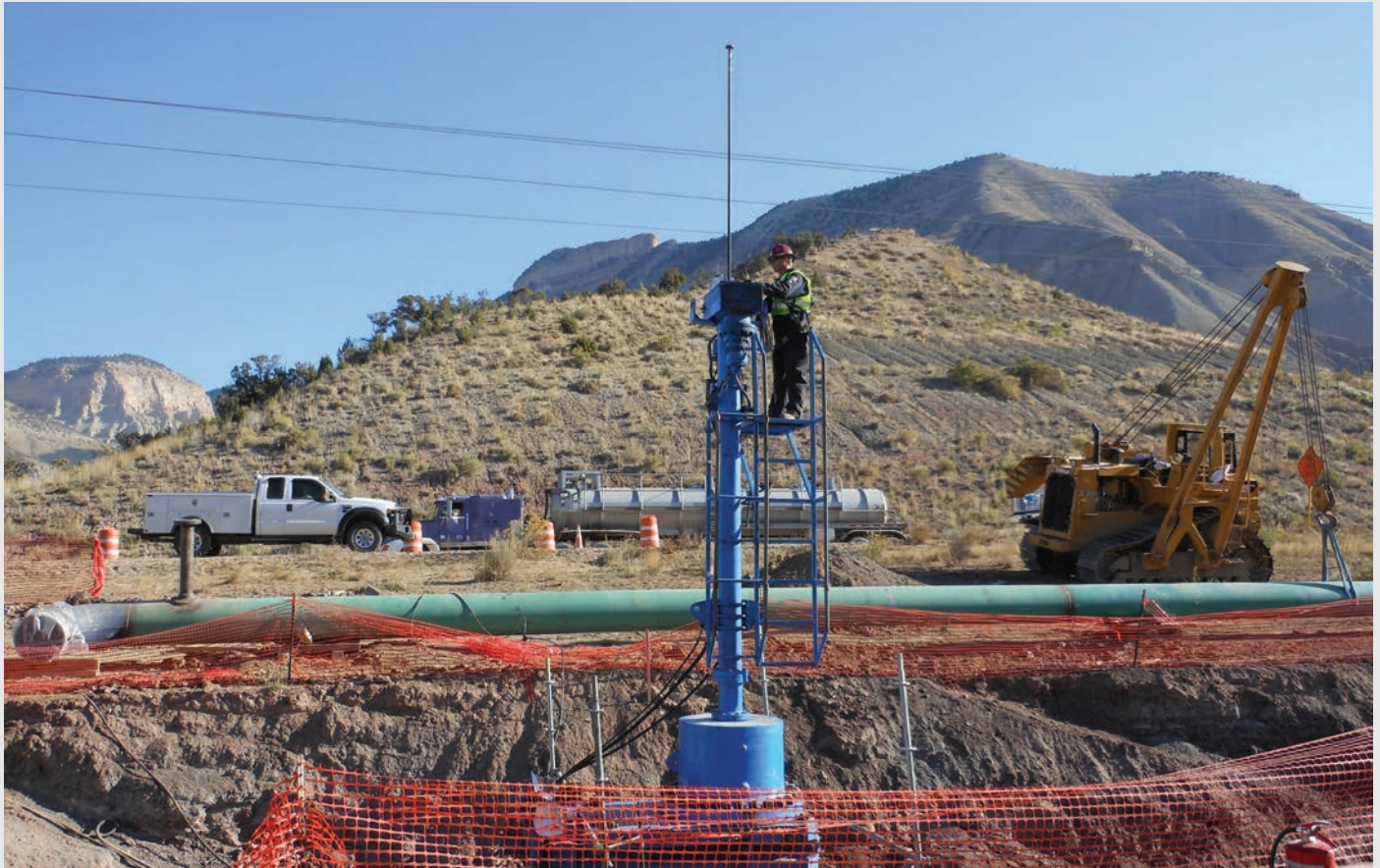
Online 400 ft. NGL Pipeline Section Replacement for Enterprise Products
