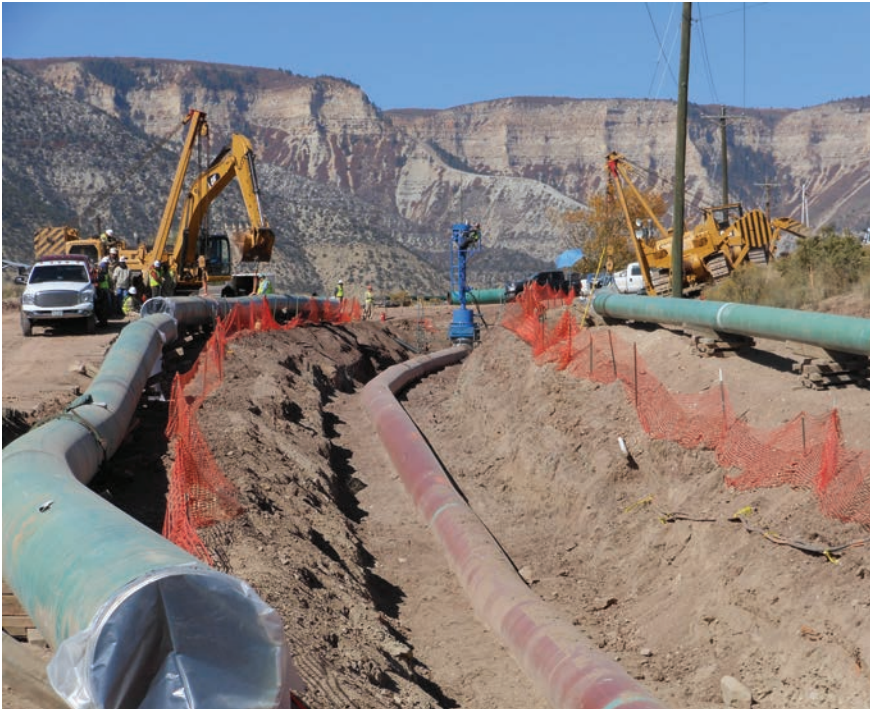
Online 400 ft. NGL Pipeline Section Replacement for Enterprise Products
