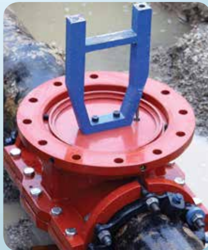
Internal equalization completion plug installed.
